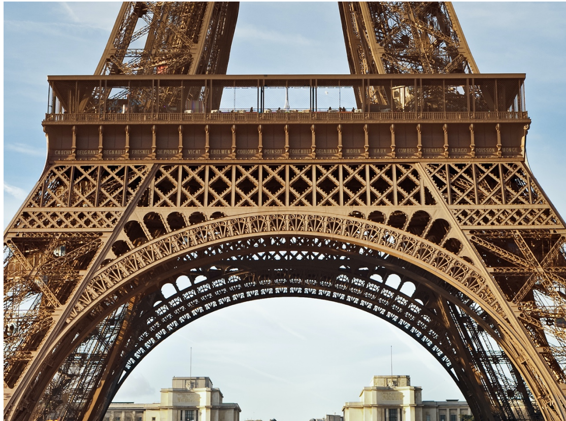
Figure 6. The arches and openwork cross-bracing of the Eiffel Tower
