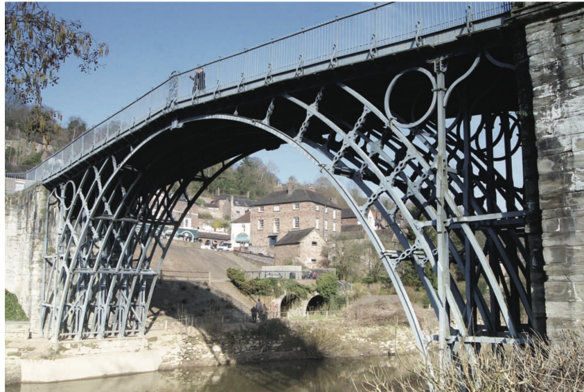
Figure 2: General view of the bridge in 2014 (Miller, 2015)
